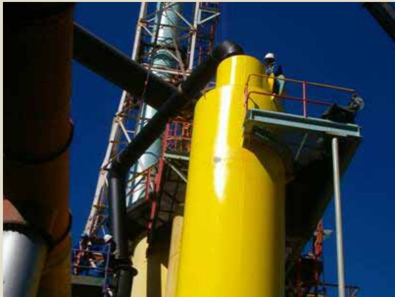
Replacement of cross flow stripper tower - 2009
