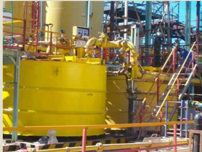
Replacement of 94% & 98% acid receivers - 2008
