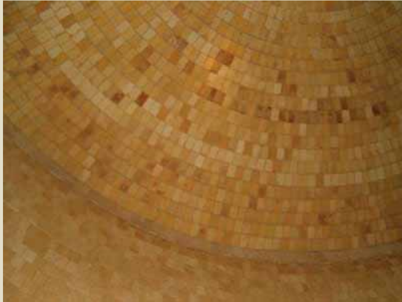
Rebuilding of No 1 roaster - 2009
