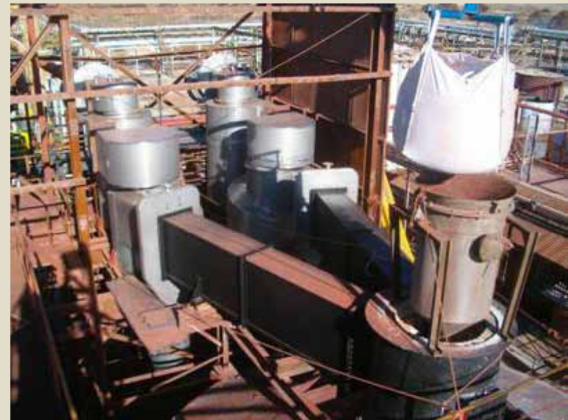
Replacement of roaster gas outlets, cyclones, square ducts and round ducts- 2008
