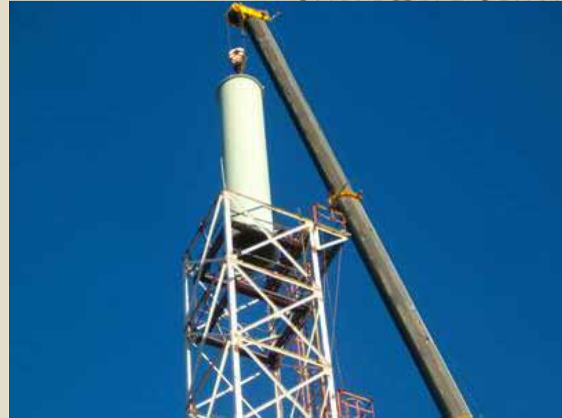
Replacement of Acid Stack - 2008
