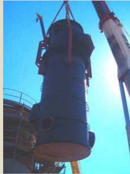
Replacement of new HHE
