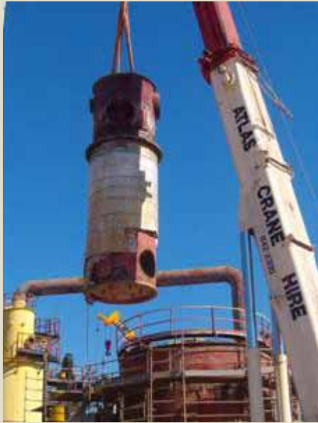
Removal of old HHE
