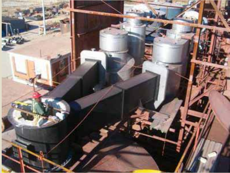
Replacement of roaster gas outlets, cyclones, square ducts and round ducts- 2008
